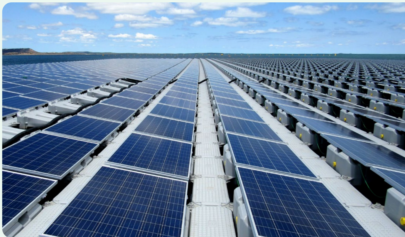
Floating solar panels on the surface of one of Chesf’s hydroelectric reservoirs. Eletrobras Chesf Archives
