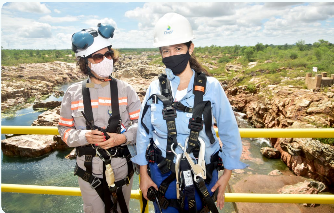
Female employees working on the main sluice gate in Algorão, at Eletrobras Chesf. Photo: André Schuler
