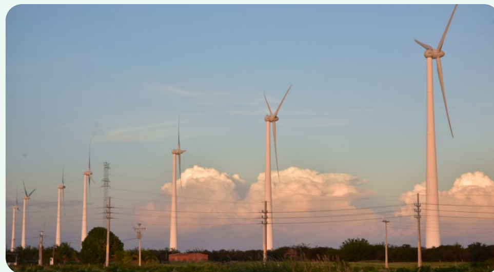
An Eletrobras Chesf wind farm. Photo: André Schuler
