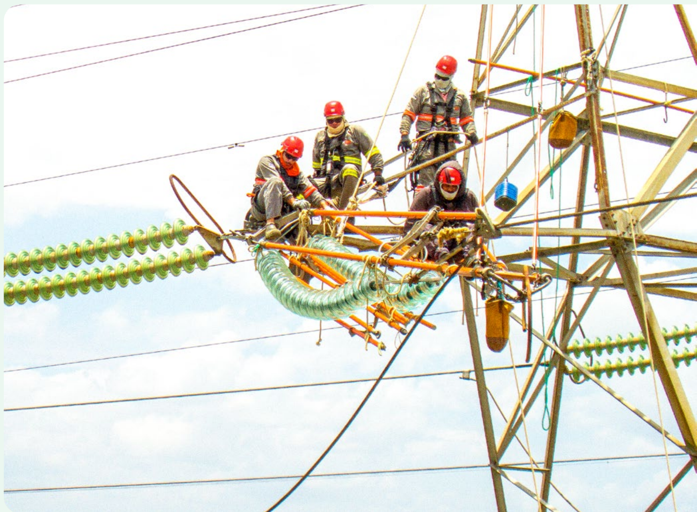
Maintenance work on an Eletrobras Chesf transmission line. Photo: André Schuler
