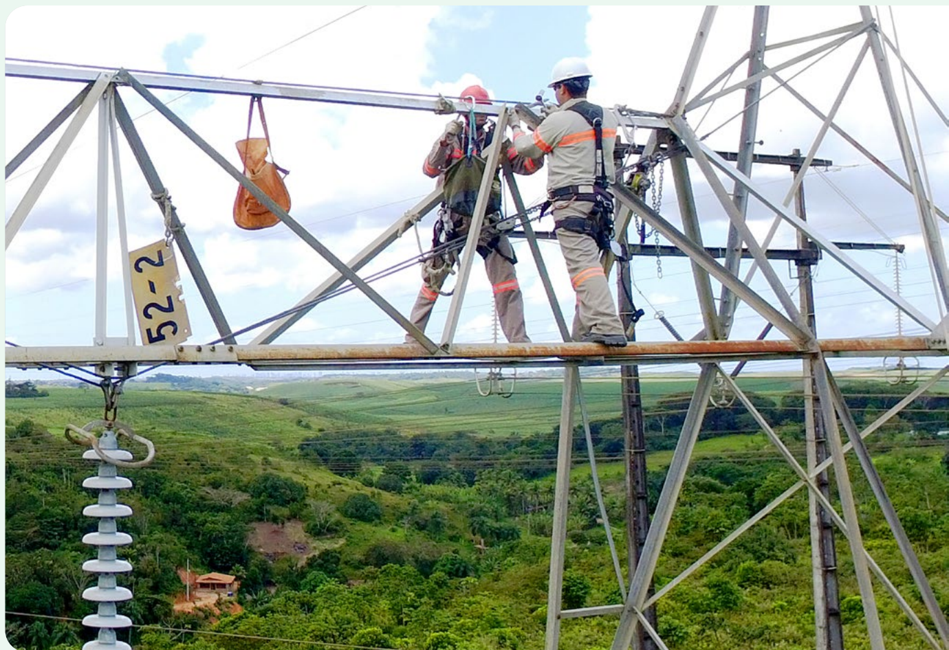
Working on a transmission line, Eletrobras Chesf. Photo: Eduardo Vilaça
