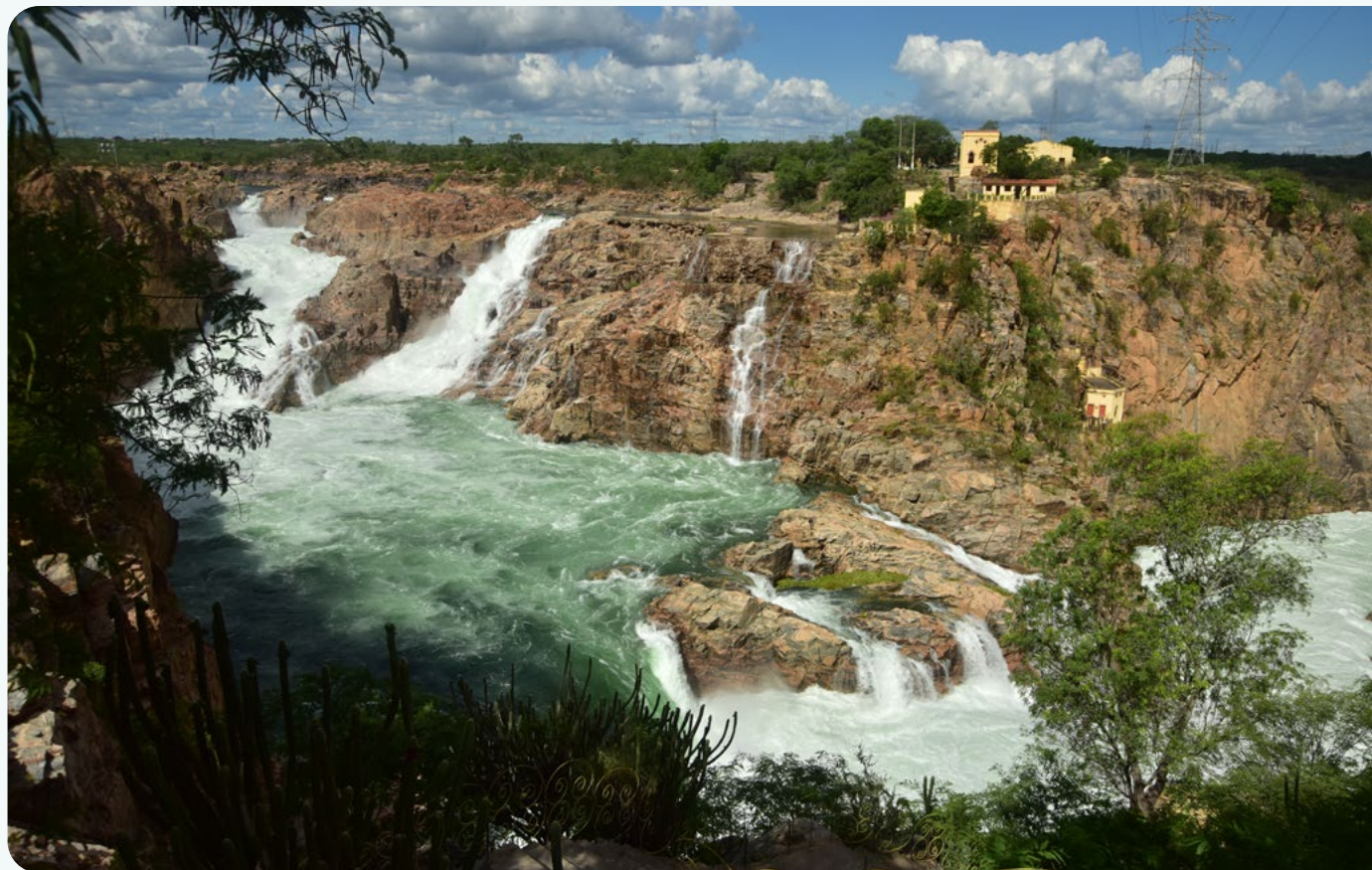
Cachoeira Paulo Afonso, Eletrobras Chesf. Photo: André Schuler
