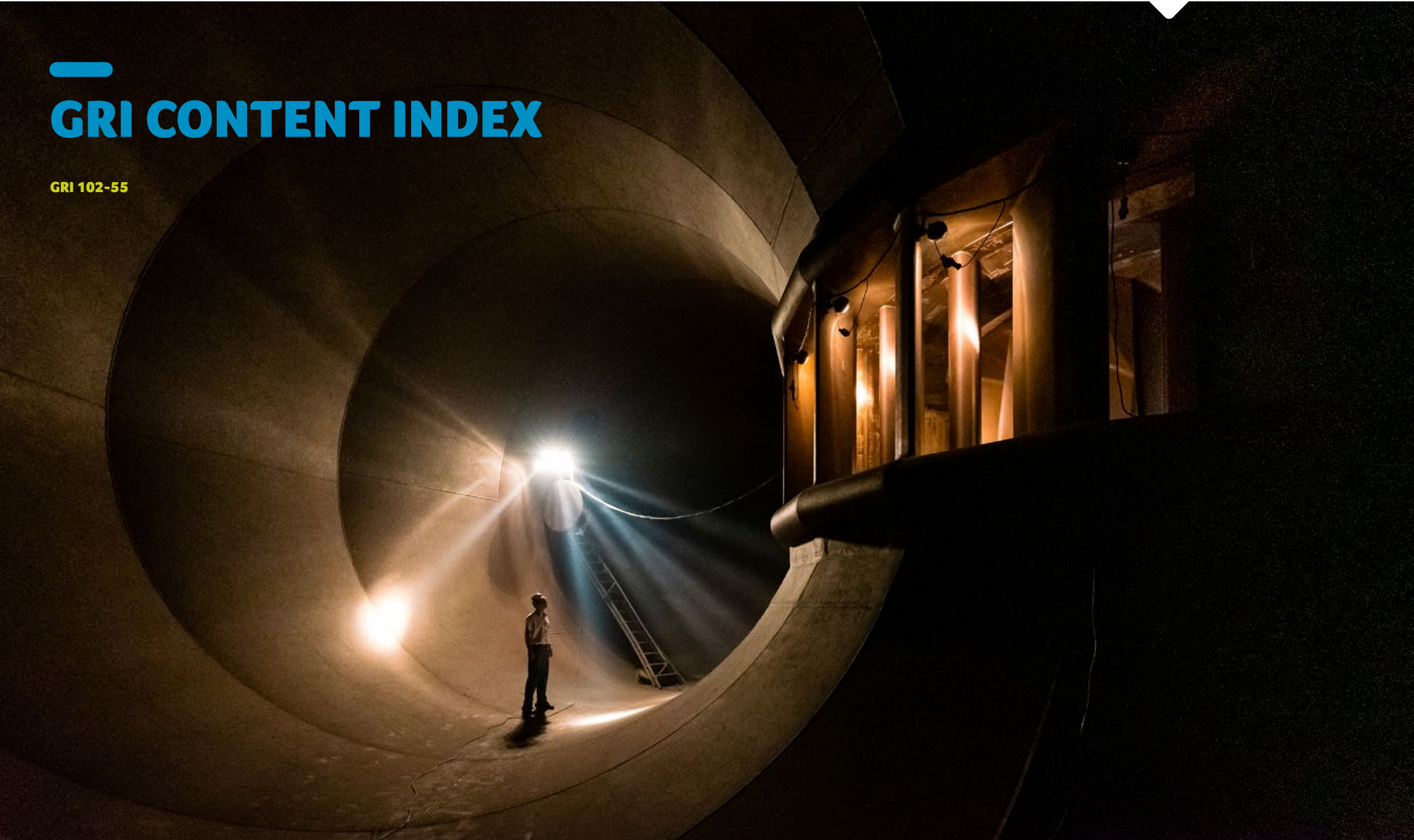
Performing maintenance work in the volute at Itaipu. Photo: Rubens Fraulini.
