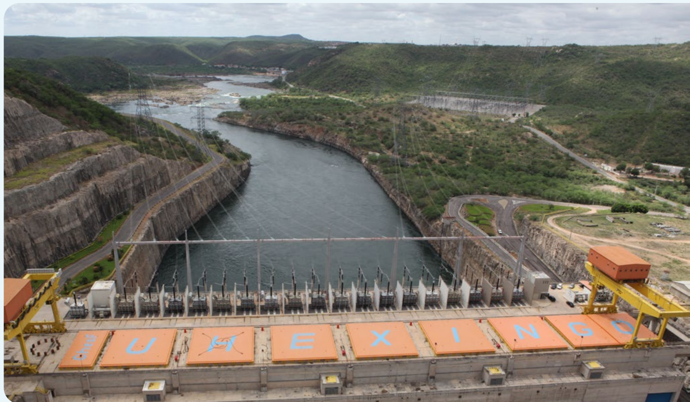
The Xingó Dam. Elétrabras Chesf Archives
