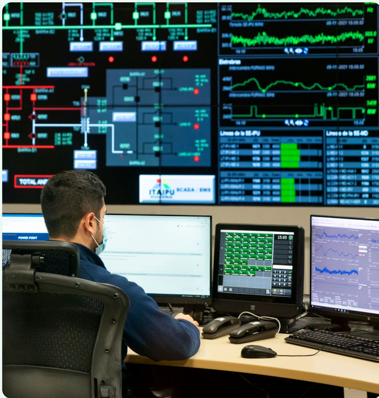
A load dispatching control room at Itaipu. Photo: Sara Cheida
